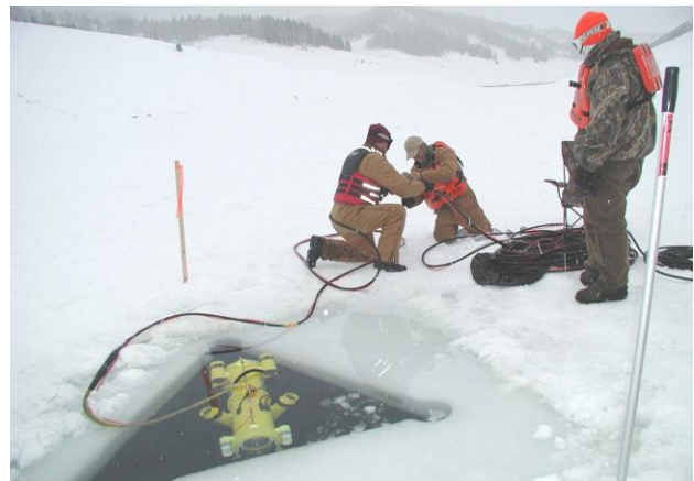
Figure 14. SeaLion Inspecting Ice-covered Reservoir
