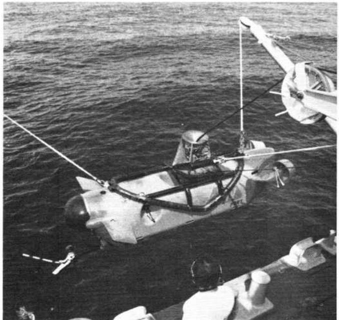
**Fig. 4** The MNV being launched during at-sea mine neutralization tests
